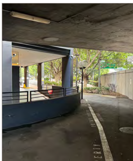
8. Under Western Distributor
