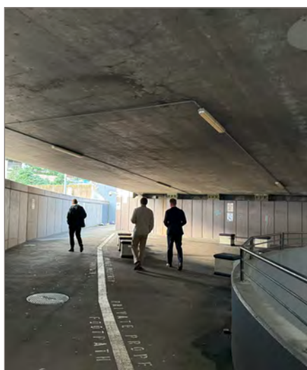
7. Under Western Distributor
